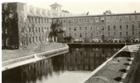
Raceway at the Wauregan Mills, c. 1950. Industrial-era aceways were wide and deep like canals and carried large amounts of water to power the mills. From the collections of the Windham Textile and History
