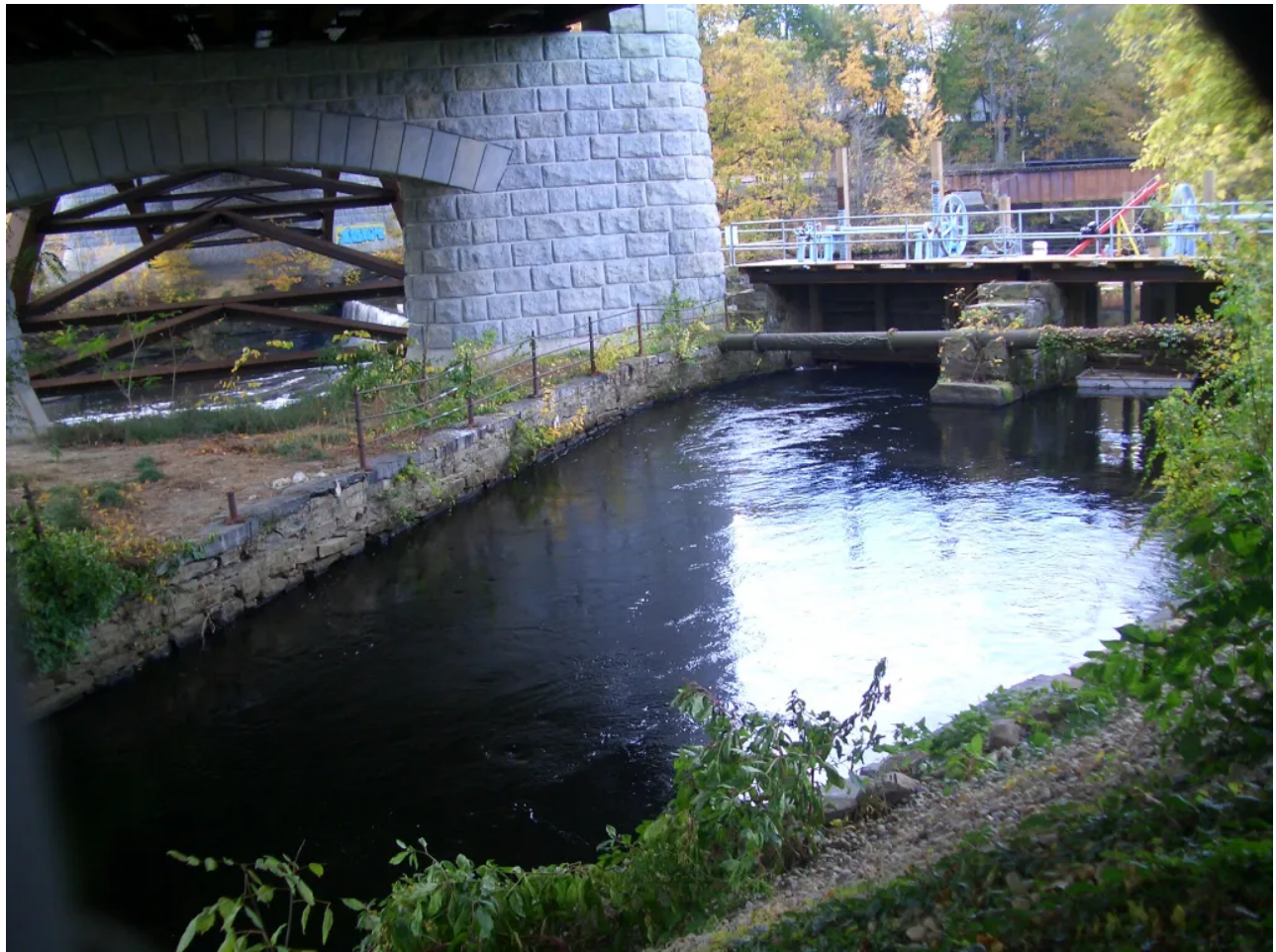
This head race (the part of the raceway that carries water to the mill's wheelhouse) flowed from the Willimantic River to the Willimantic Linen Company's Spool Shop and Mill No. 1. Sluice gates (shown upper right) controlled the amount of water entering the raceway. The sewer pipe, railroad bridge, and stanchions of today's Frog Bridge for vehicular traffic were added later. Today, the water in the raceway turns turbines that generate electricity. From the collections of the Windham Textile and History Museum. Photo by Stephanie Conforti.
