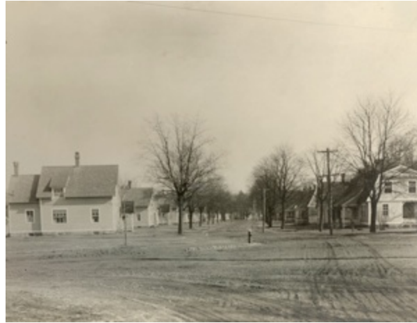
The Oaks, a neighborhood of quaint, six-room, freestanding Victorian cottages that William E. Barrows, the General Manager of the Willimantic Linen Company in Willimantic, Connecticut, had built for his workers in the 1880s. Photo c. 1880, from the collections of the Windham Textile and History Museum.
