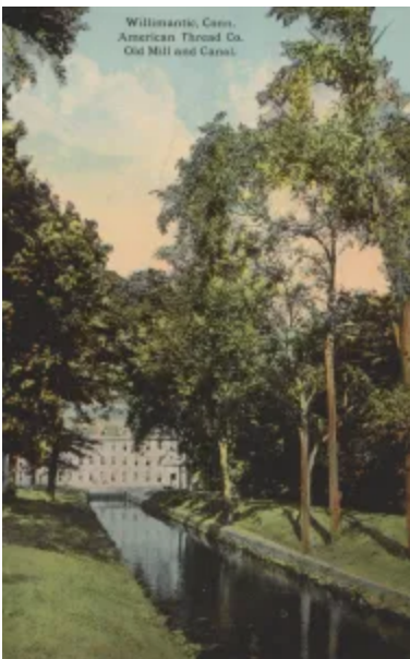
Raceway (canal) leading to Mill #3 (the former Richmond mill), c. 1905. From a postcard in the Mill Museum collection.
