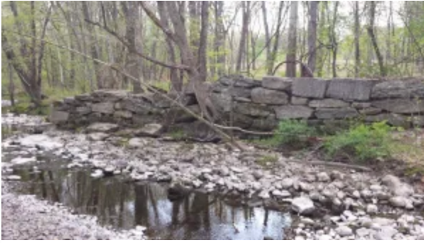
Remnant of Richmond mill dam, south bank of the Willimantic River (opposite bank from the mill). The top layer of quarry stone may have been added later. Photo by Jamie Eves.
