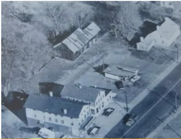
Aerial photograph of part of Down Sodom c. 1960s, showing Main Street. The house at the top right is the Carpenter cottage, built in the early 1800s by Lorin Carpenter and owned for most of the 19th century by John Capen.
