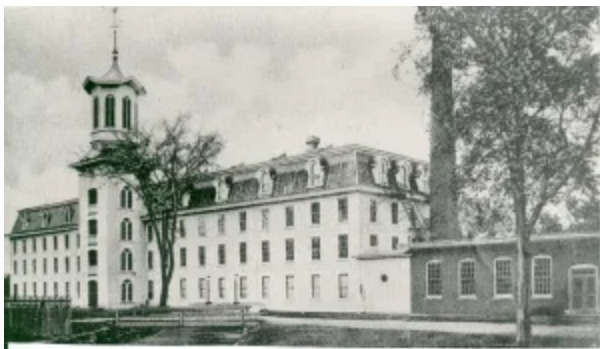
The Welles or Dunham mill, built in 1845 by Lloyd Baldwin. It was renamed Mill #3 when the Willimantic Linen Company acquired it. Photo from the Mill Museum collection.
